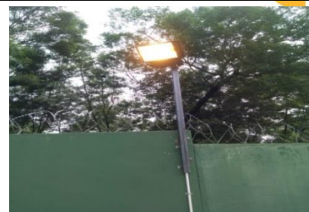
Repairs of lights at Truck Entrance
