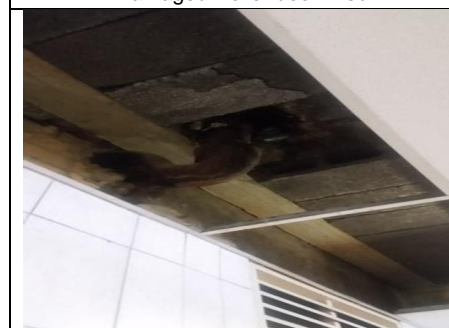
Sewer Pipe@ 5 th Floor Fixed
