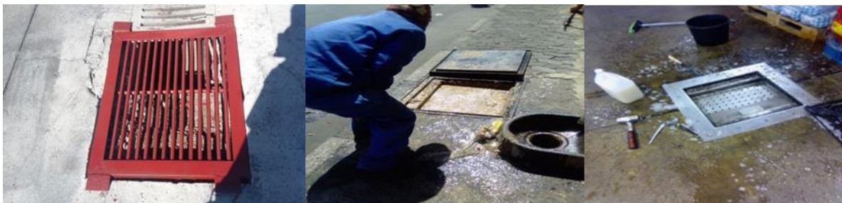
Cleaning & Unblocking of Drains
