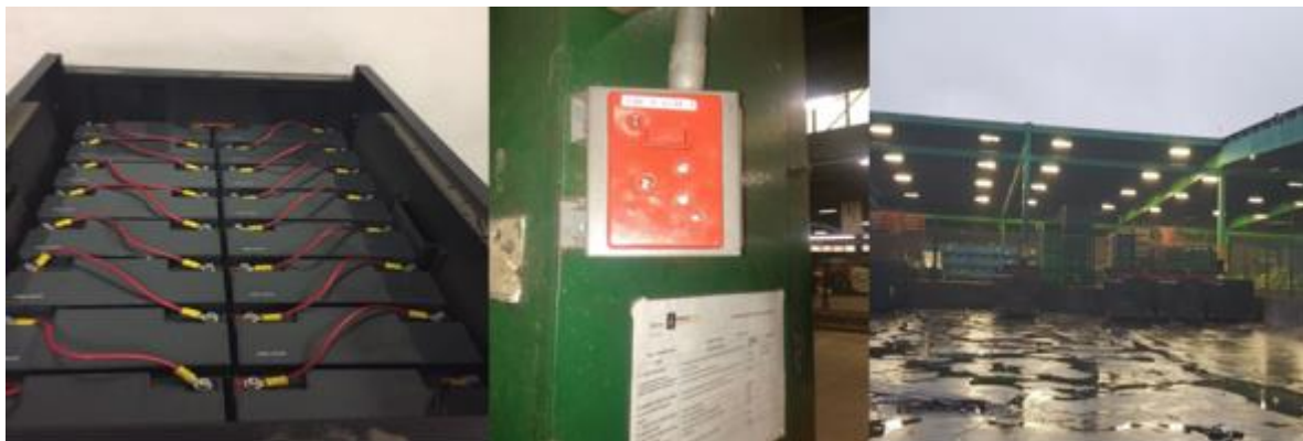
UPS, Plugs & Lights Repairs
